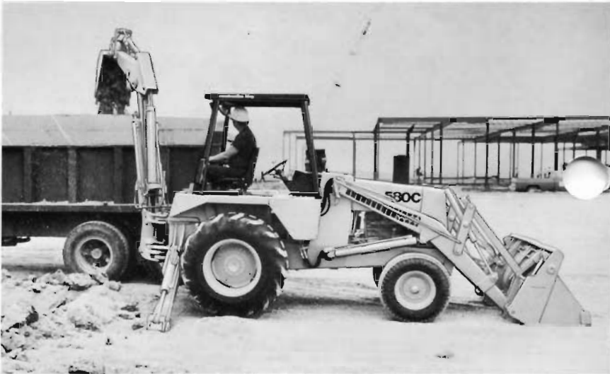
14' (4267 mm) backhoe speeds excavating and truck loading cycles.
